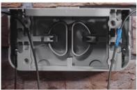
Unwrap the cable <u>removing any twists</u> (if necessary tape to wall)
