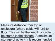
Prepare the route for the cable length from start to finish allowing correct length for each Façade closure.
