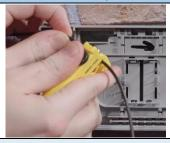
Using 'Adjustable Ring and Slit Stripping Tool for BFT Interception (Yellow Peg) 112794', cut a 50-100mm (2-4") window approximately 50mm from the Entry P Clip
