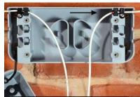
Unwrap the cable <u>removing any twists</u> (if necessary tape to wall)
