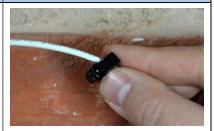
• Place the first 'P' Clip over the entry side of the feeder cable.
