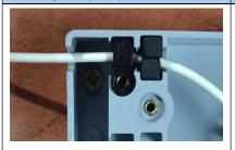
Slide on the split seal over the feeder cable
