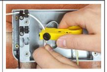
Using 'Adjustable Ring and Slit Stripping Tool for BFT Interception (Yellow Peg) 112794', cut a 50-100mm (2-4") window approximately 50mm from the Entry P Clip
