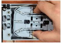
Wrap the marked length around the outside of the tray mandrel so the tape or reflective pen are on the inside of the second seal position.
