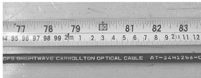
Figure 23 - Measure and mark the mid-span sheath opening
