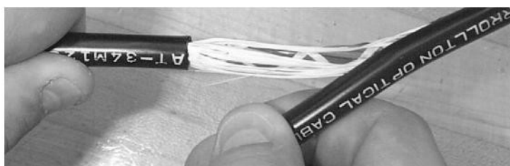
Figure 7 - Remove the outer sheath
