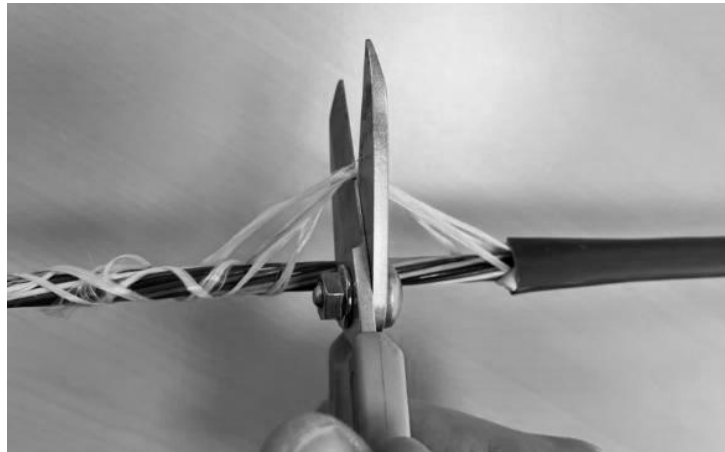
Figure 27 . Remove and cut the binder threads
