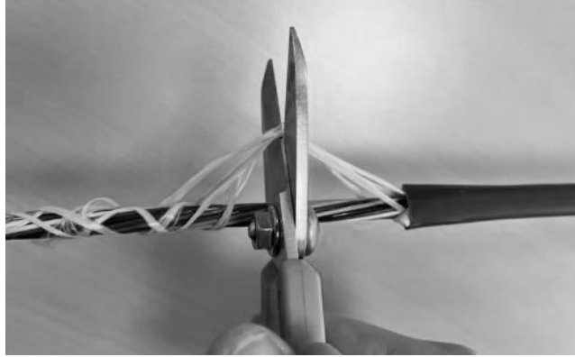
Figure 8 - Remove and cut the binder threads
