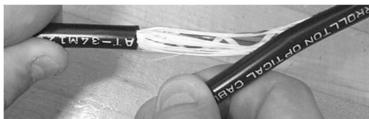
Figure 7 - Remove the outer sheath
