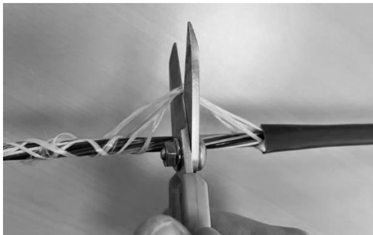
Figure 27 . Remove and cut the binder threads
