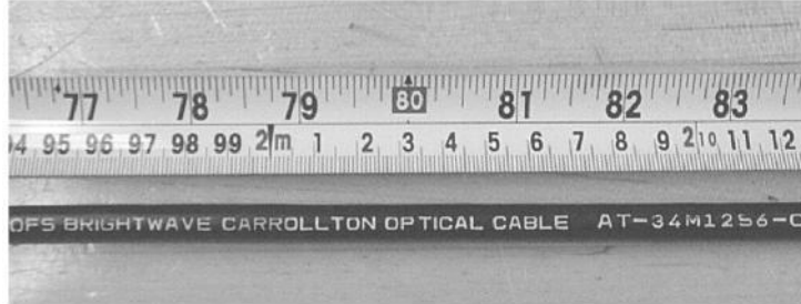
Figure 16 - Measure and mark the cable.
