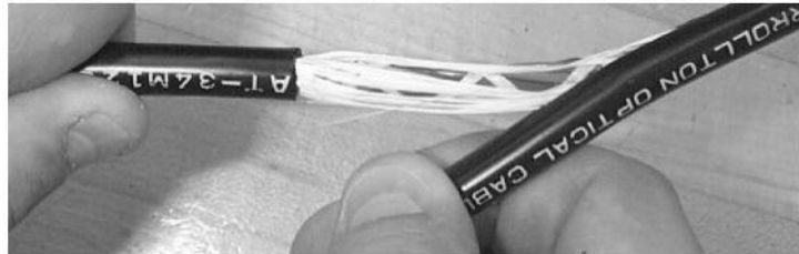
Figure 20 . Remove the 300mm section of outer sheath
