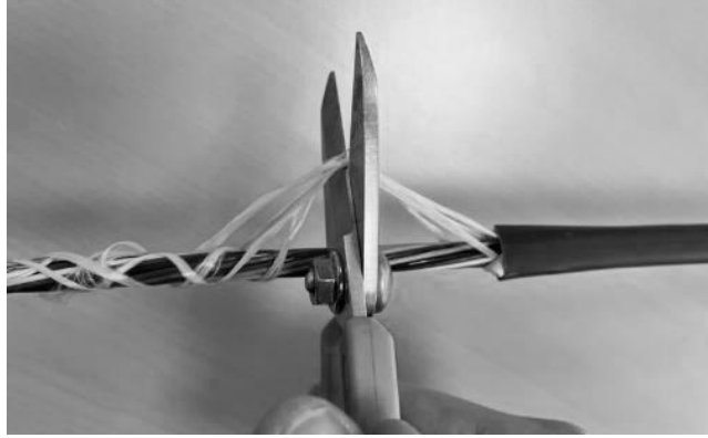
Figure 8 - Remove and cut the binder threads
